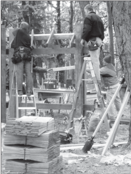
(At left) Experienced volunteers build the kiosk
